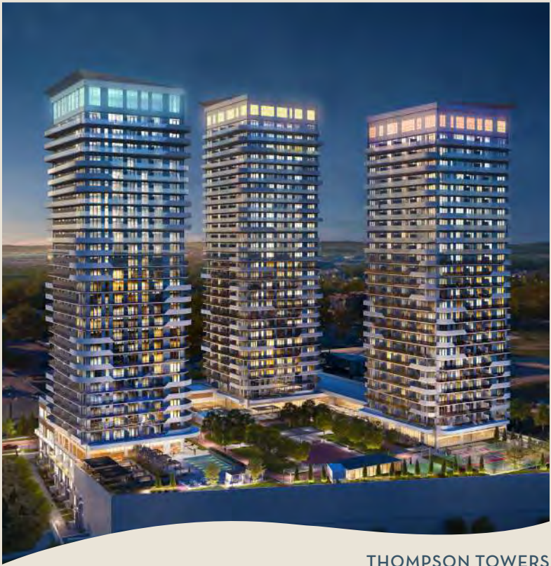
THOMPSON TOWERS MILTON
